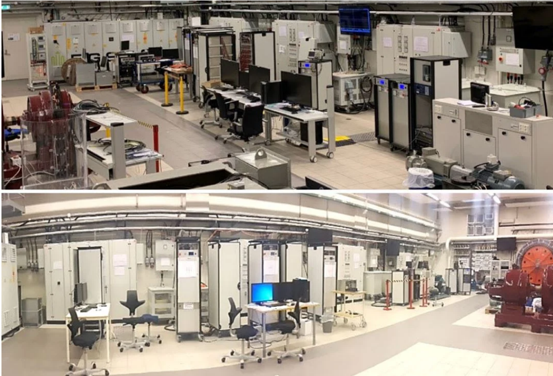
Figure 21: Picture of the National Smart Grid Laboratory [92]
