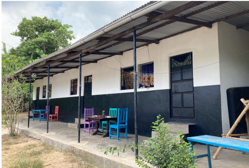
Figure 17: The outside of the Staff Court at Eco Moyo.
