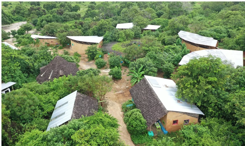
Figure 12: Overview of The Staff Room and Classrooms at Eco Moyo [62, p.44].
