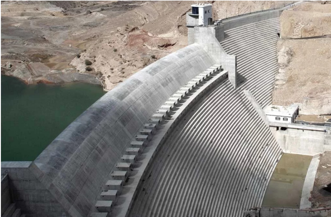
Figure 2.2.1: Wadi Dayqah main dam, Oman (CCC 2009).
