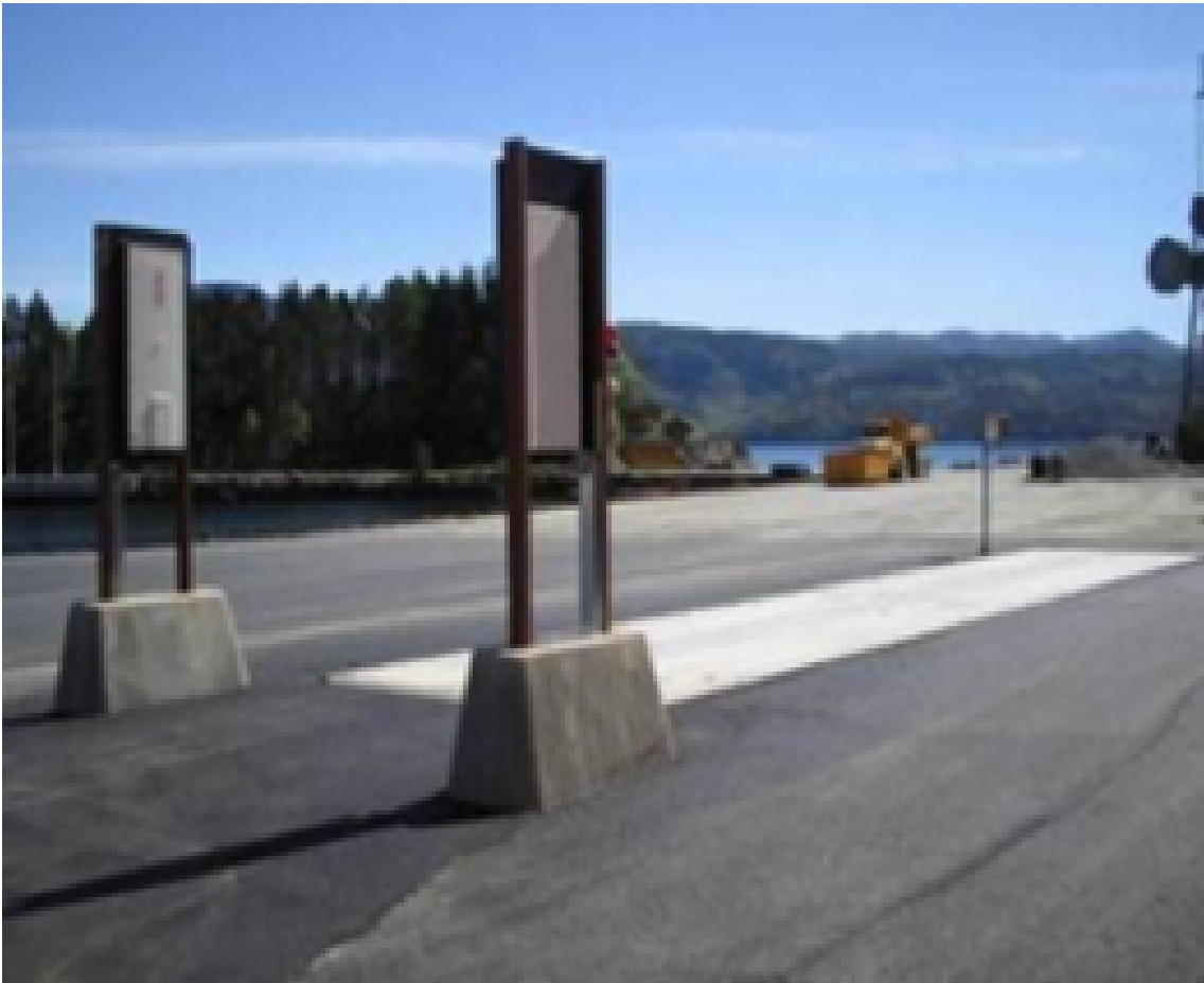
Figure 9: Weight and NORM Radar (Internal Source with Permission from AF Offshore Decom)
