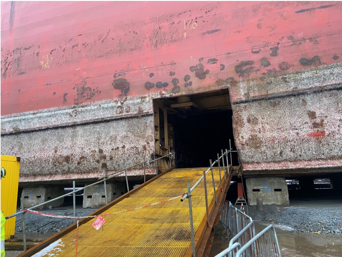
Figure 6: Opening to Entry Lifts for Washing (Internal Source with Permission from AF Offshore Decom)
