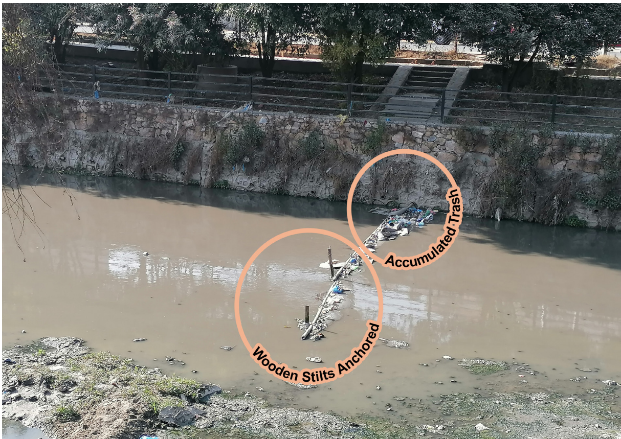
Fig 68. Wooden poles retaining floating trash in Aloknagar District (Source: Author, 2023)
