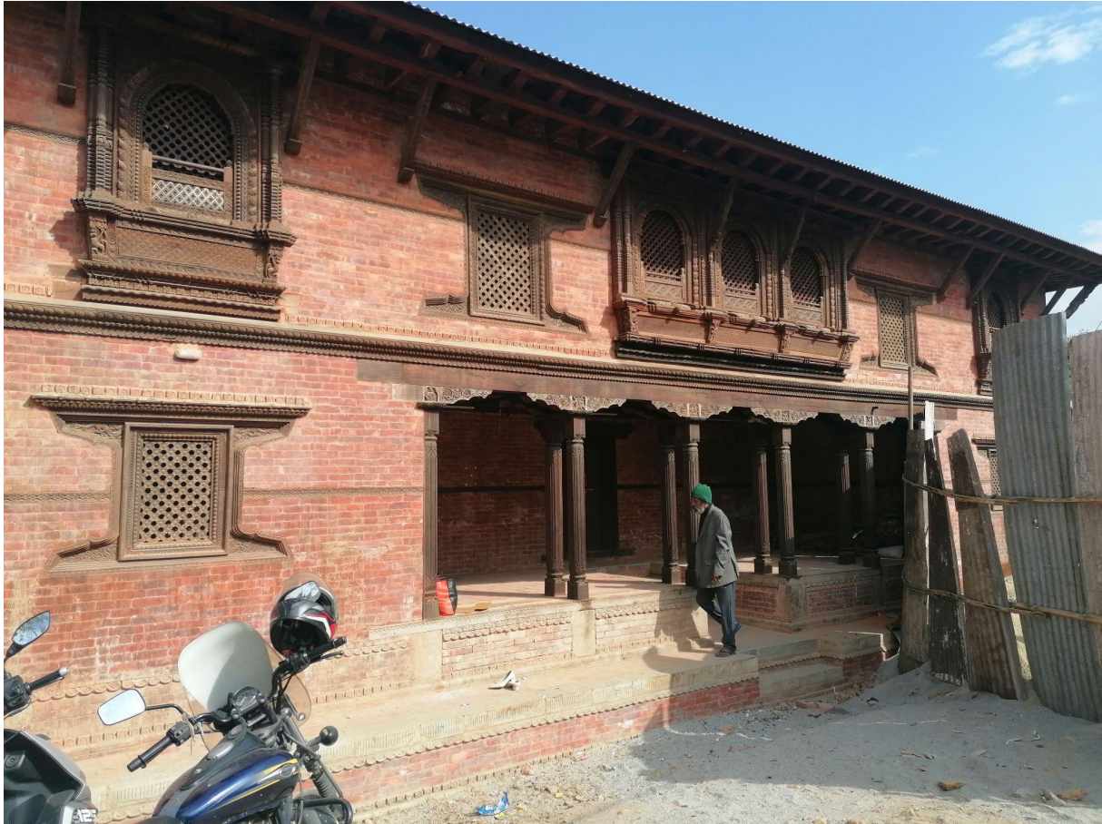
Fig 42. Restoration of Mokshya Dhaam temple Tripureshwor District (Source: Author, 2023)
