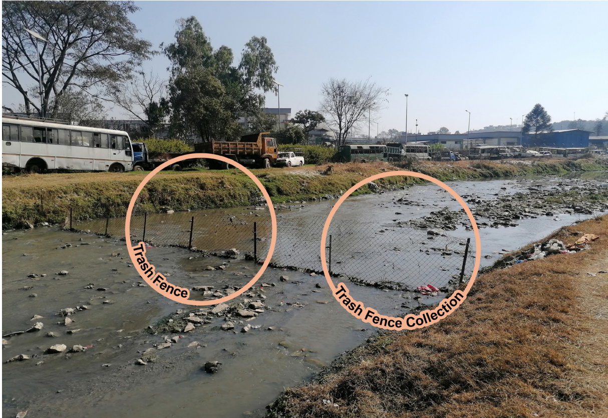
Fig 67. Retaining fence found in Bagmati River near Pashupatinath Temple (Source: Author, 2023)
