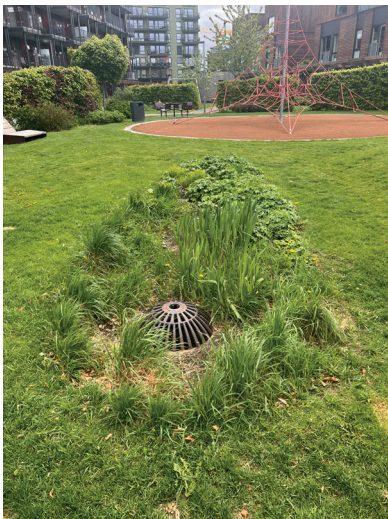
Figur 37: Regnbed for overflatevann
