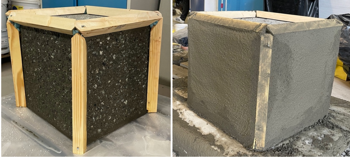
Figure 5-8: Concrete repair: Before (left) and after (right) dry shotcrete repair with Dry shotcrete Sprøytetep T
