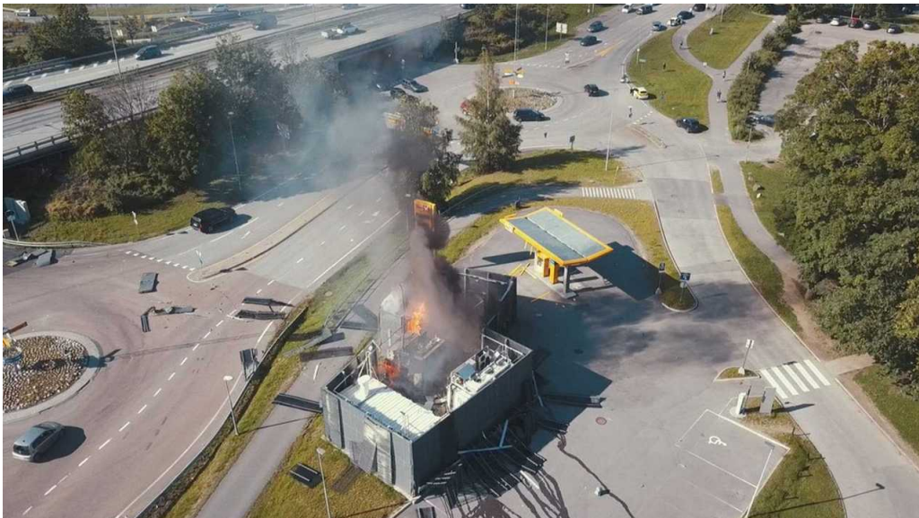
Figure 1: The Sandvika hydrogen refueling station [35]
