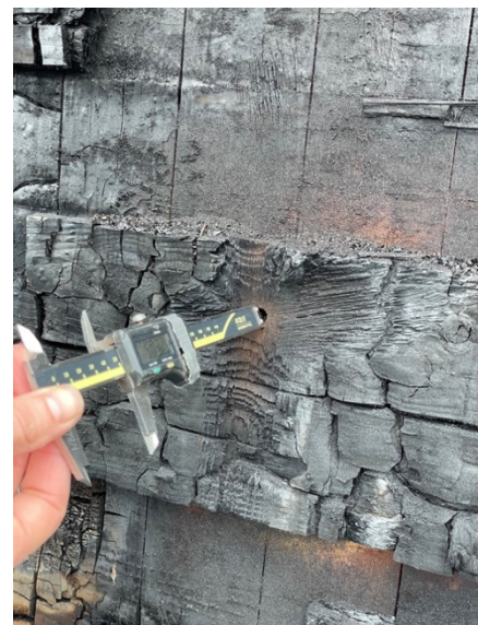
Figure 2.4 Caliper used to measure charring depth from ceiling elements used in the Compartment Test.
