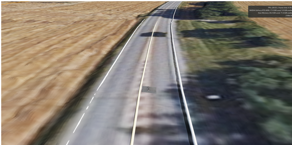
Figure 4.16: Potential visualization of cracked road in our digital twin
