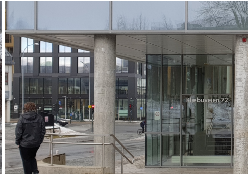
(c) Corner, looking west
