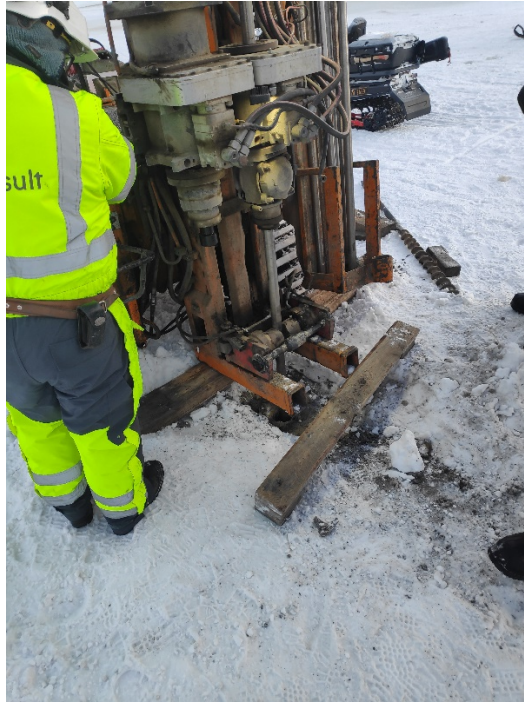
Figure A.3 UNIS East – Multiconsult drilling
