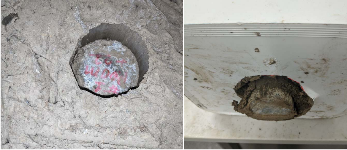
Figure A.23 Failure mechanism of stage 1 #1 sample: left (a) – adfreeze shear along the soil well, and right (b) – concrete cylinder out of the designed bucket hole
