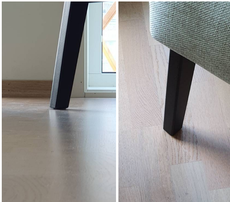
(a) Glossy reflection when viewed from a low angle. (b) No glossy reflection when viewed directly from above.
