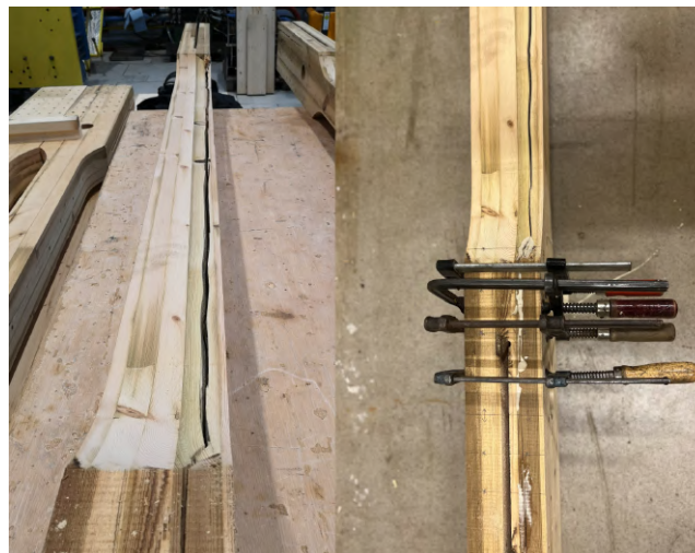
Figure 16: Application of wood glue to the longitudinal cracks in S4 .
