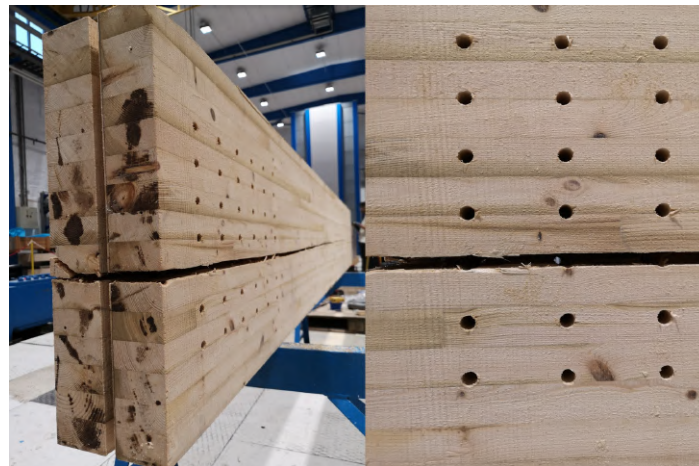
Figure 23: Horizontal crack in B2 that weakens one dowel row.
