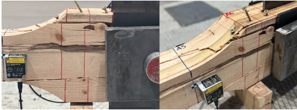
Figure 35: Failure of S4.
