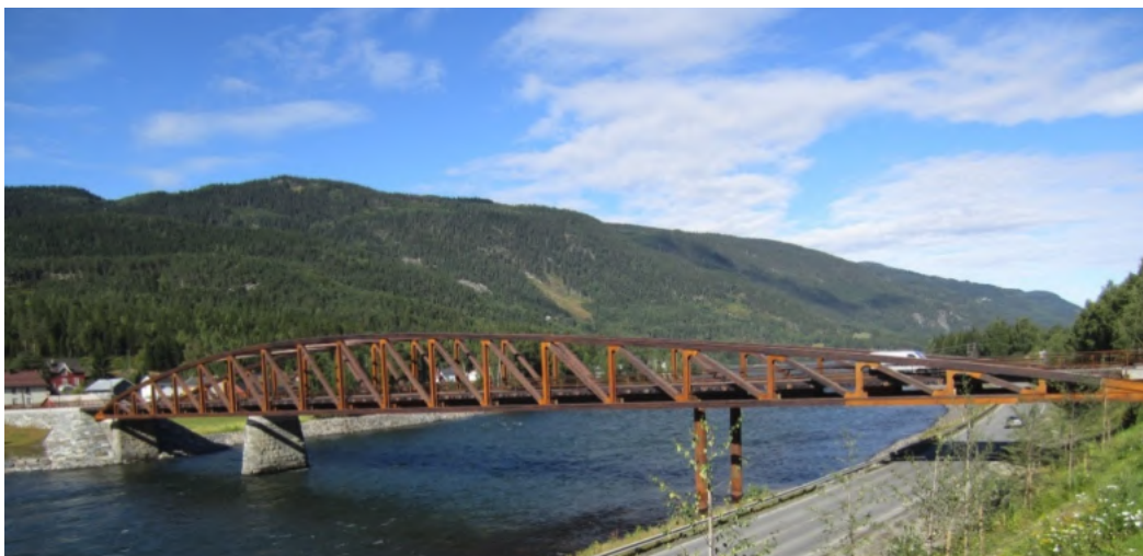
Figure 17: The new Tretten bridge opened for traffic in June 2012 (Hårstad-Evjen et al. 2013a).
