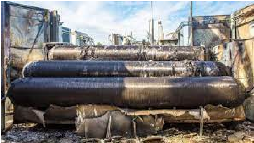
Figure 8: Tanks of the refueling station of Kjorbo
