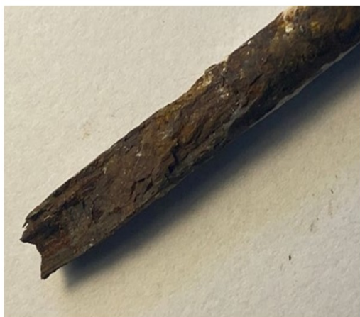
(a) Broken wire
