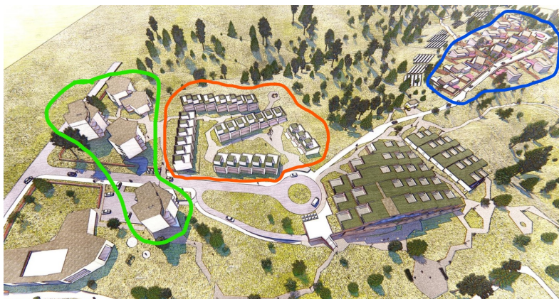
Figure 4.2: An overview of the residential area[49].
