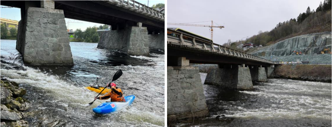
Figure 4: Sluppen bridge from the downstream side (picture provided by NTNU).
