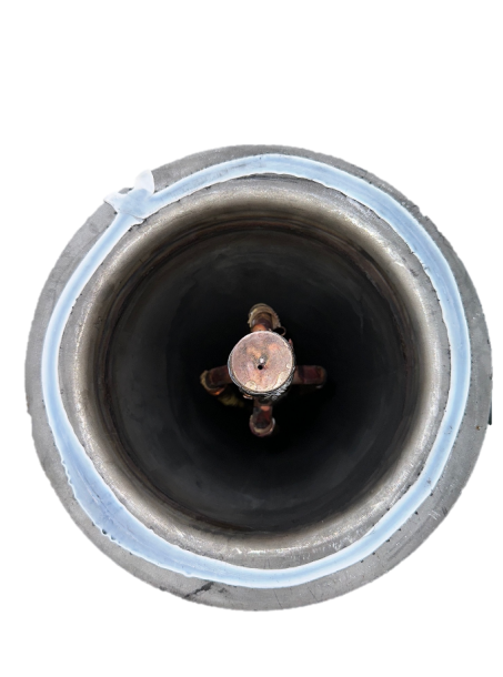
Figure 8.14: End of collector before the flange is mounted.
