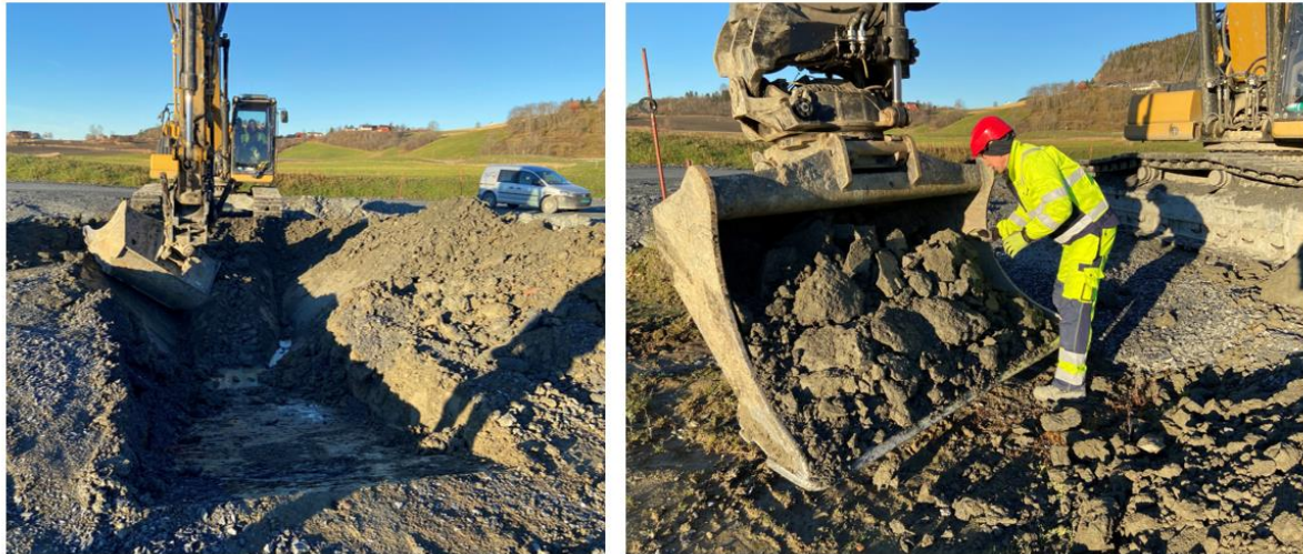
Figure 26: Collecting MDM samples using an excavator.
