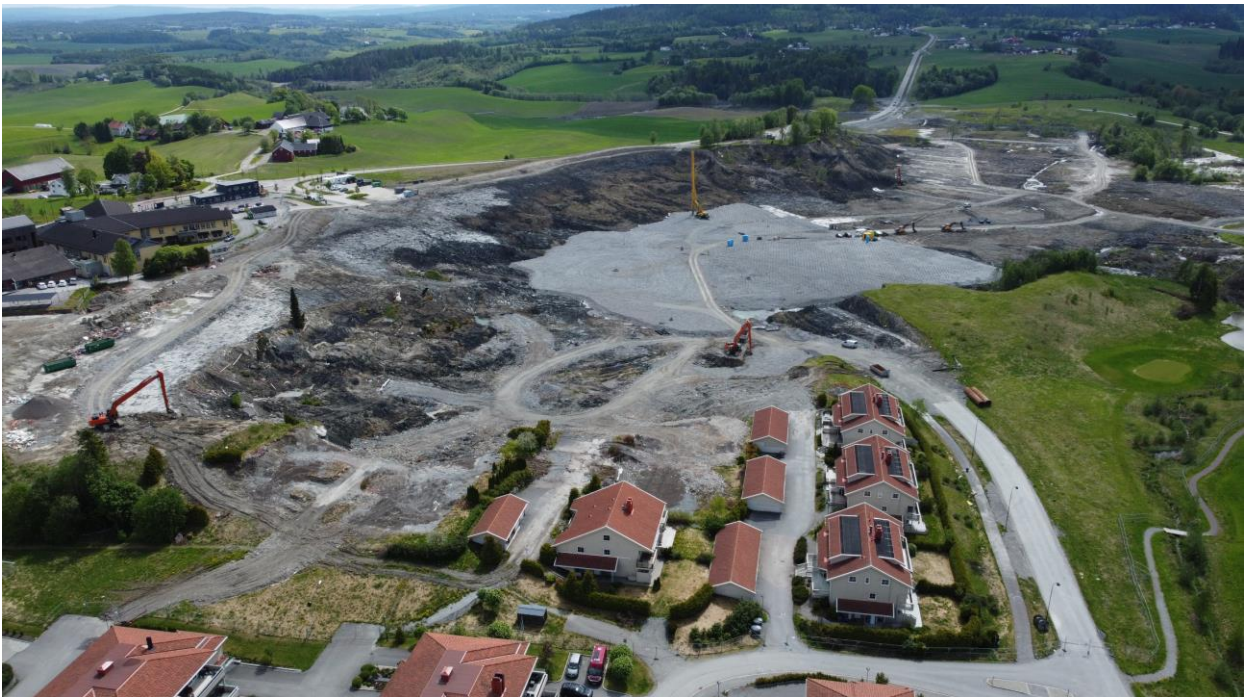
Figure 16. Dronephoto: 30.05.22. The terrain is relieved at the northern edges. Photocredit: Gjerdrum kommune
