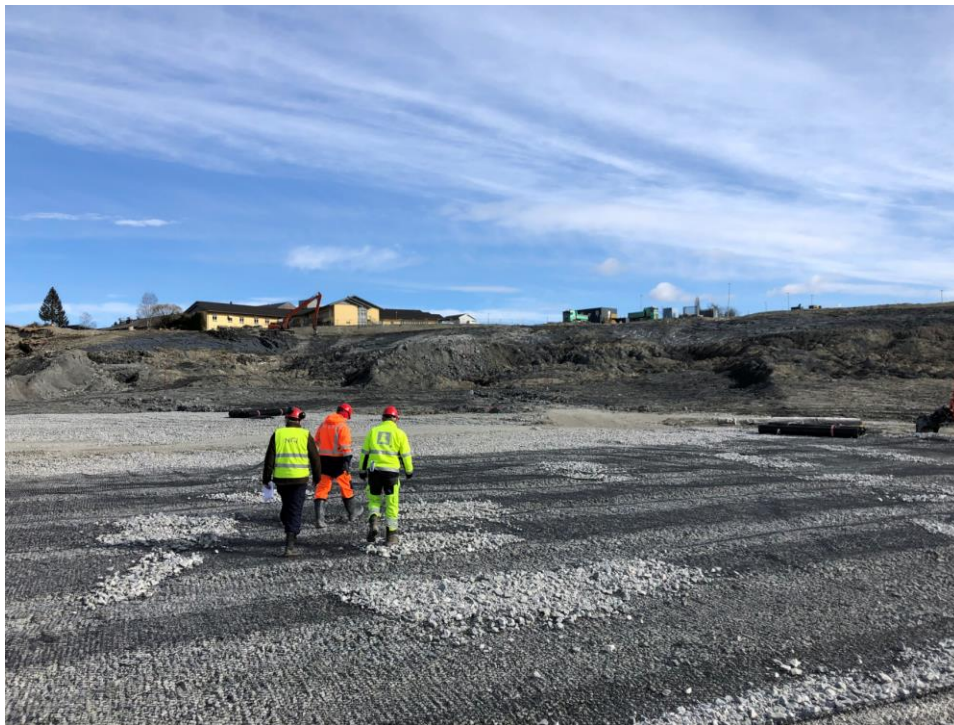
Figure 14. Inspection 29.03.22. Terrain is smoothed out with gravel on top. Photocredit: NGI
