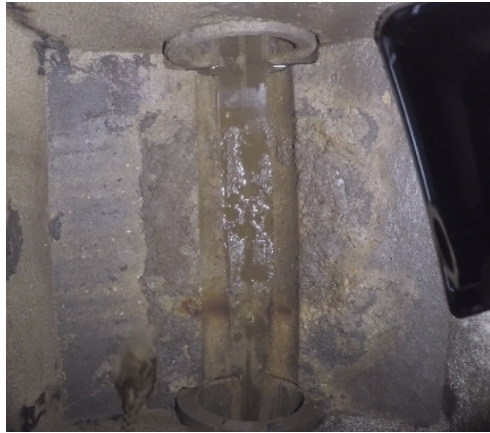
Figure 5.7: This camera view is optimal for the purpose of optical velocimetry implementation in sewers as it can capture the entire flow field. Captured with a GoPro (4K resolution).
