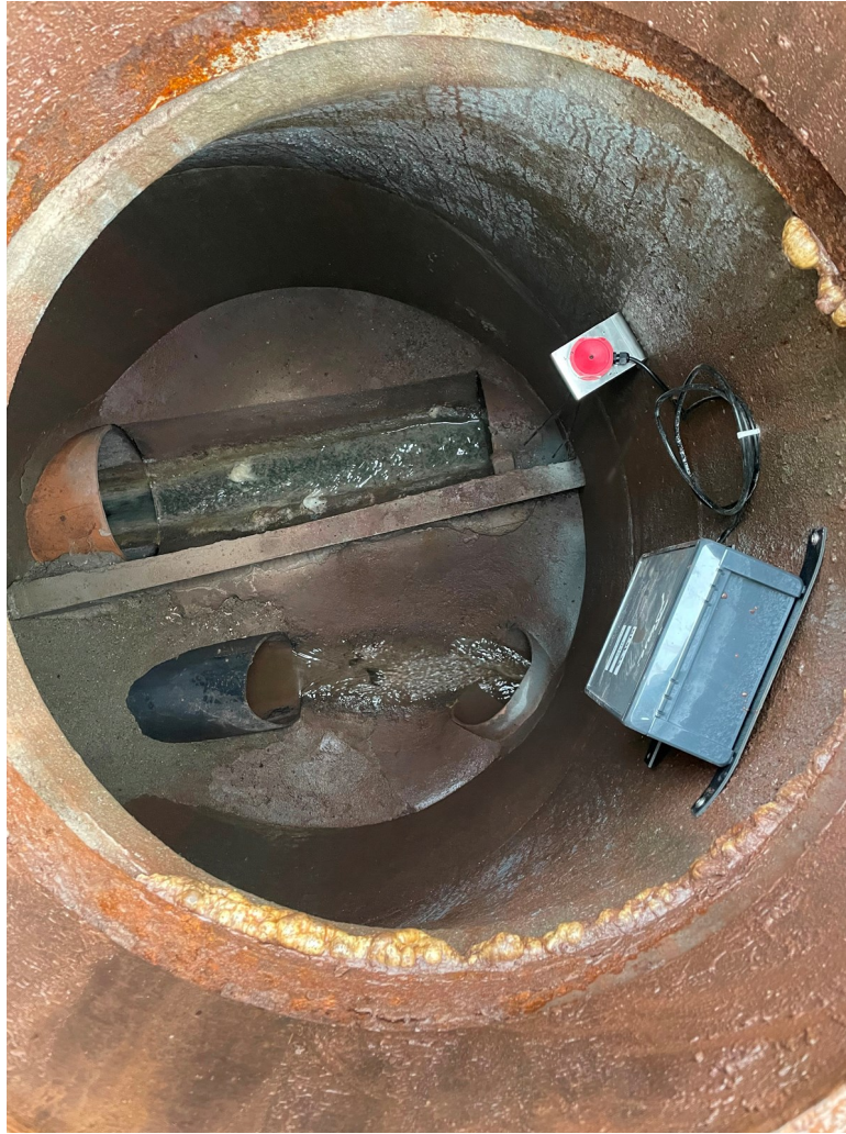
Figure 3.3: Intentional Overflow in Separated Sewer
