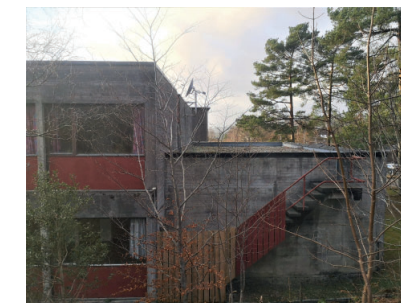
TAK OVER AUDITORIUM
