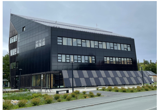
Figure 5.2: The ZEB Laboratory seen from the southwest.
