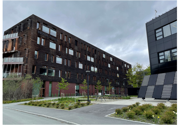
(d) The Nina building placed to the west of the building.
