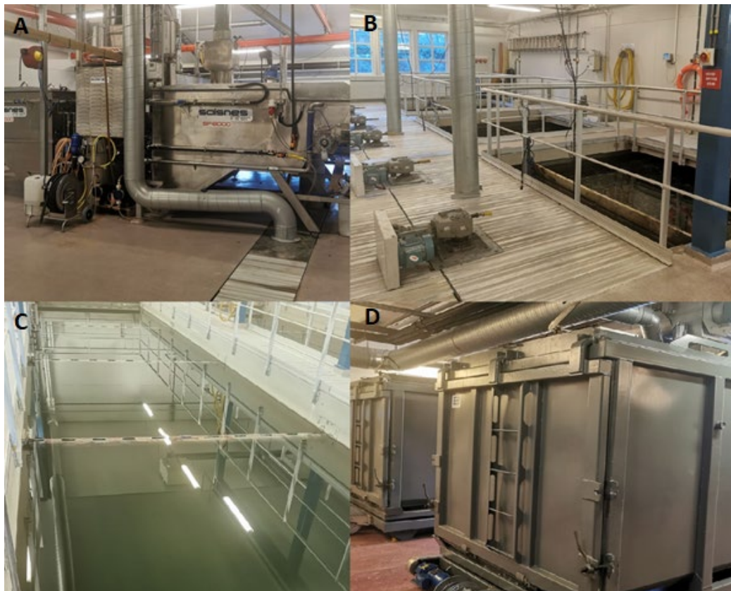
Figure 12. Pictures from site visit, A) mechanical screening, B) coagulation and flocculation, C) sediment basins, D) sludge containers
