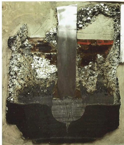
Figure 13. Recreated cross section with various materials (top) and a picture of the cross section (bottom) from Myrhaug's pilot scale excavation, used with permission from [28]
