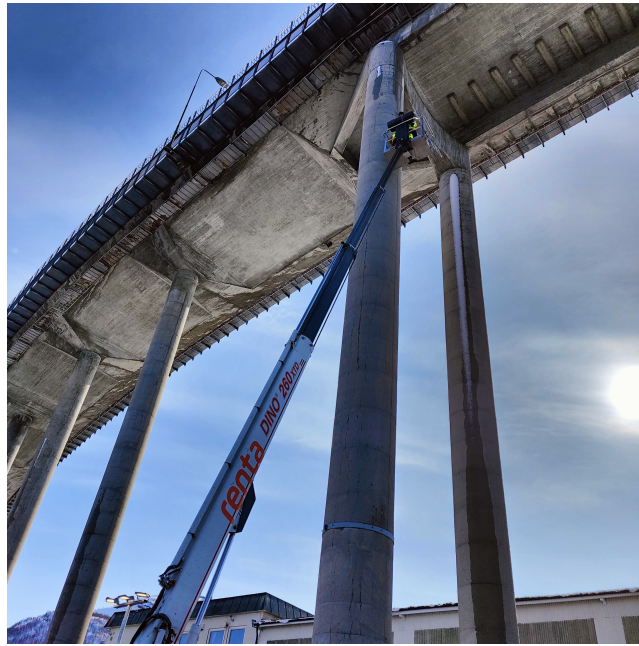
Figure 5.2: Inspection and measurements from portable lift
