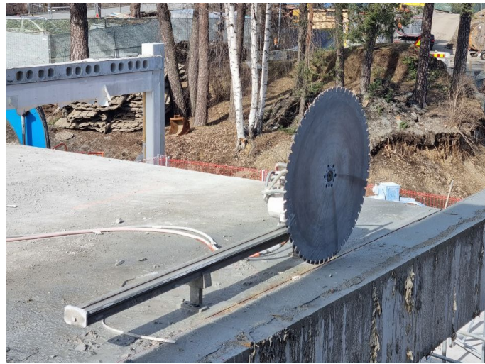
Figure 4.2: Concrete saw on rails cutting the short edge
