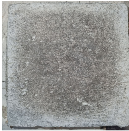
Figure 6.5: Surface of specimen applied FW324. Oily and slippery surface
