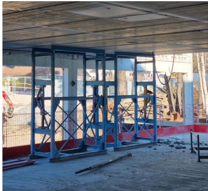
Figure 4.1: Builders trestles placed in the floor below the relevant HCS
