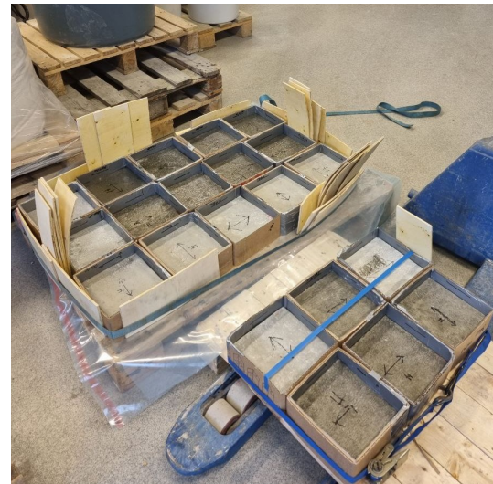
Figure 5.12: Formwork after leveling and tightened with a ratchet strap
