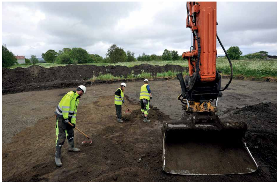
Figure 3. Top-soil stripping before and now: Same method, different attire. A) Trønd Løken following the excavator at Forsandmoen, Western Norway in the 1980s. Photo ©CC BY-NC-NC, Digitalmuseum.no. B) Tharald Bull Strømnes, Ingvild Grønbeck and Eystein Østmoe following the excavator at Ørland, Central Norway in 2015. Photo: Åge Hojem, NTNU University Museum.
