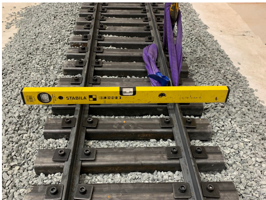
Figure 3.25.: Leveling the track with a spirit level
