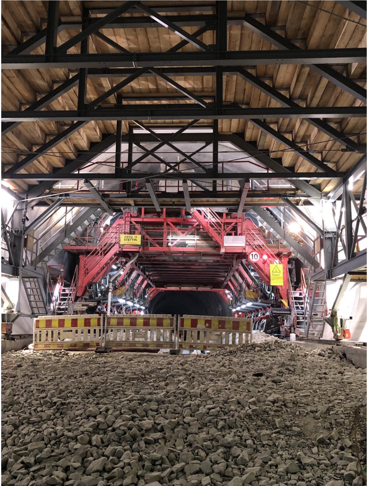
Figure D.2: Picture of the permanent lining being cast, 28.11.2022.
