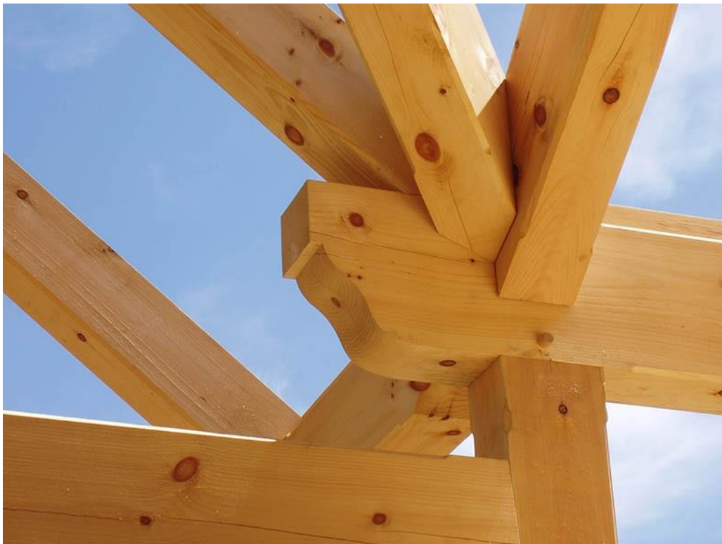
Figure 10: Knots at the timber construction (Beam, 2023)
