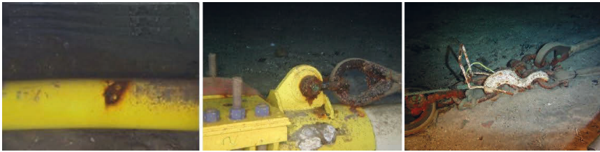
FIGURE 2.10. Example of external corrosion on subsea pipeline and pipe equipment 25 © Anonymous Operator
