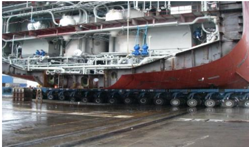
Figure 5: Prefabricated, painted block with installed pipe systems.
