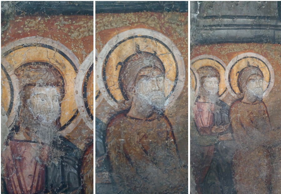
Figure 2.5: Discernible retouching (impressionistic hatching) examples at Kretzulescu church, Bucharest (external wall, front entrance), visualized from different distances. The inpainted areas are meant to make the lacunae look less disruptive from far away, as spatial mixing occurs. At the same time, from up-close, every line in the hatching is supposed to be distinguishable.
