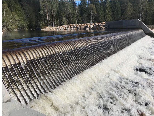
Figur 9: Coanda-inntak [38].
