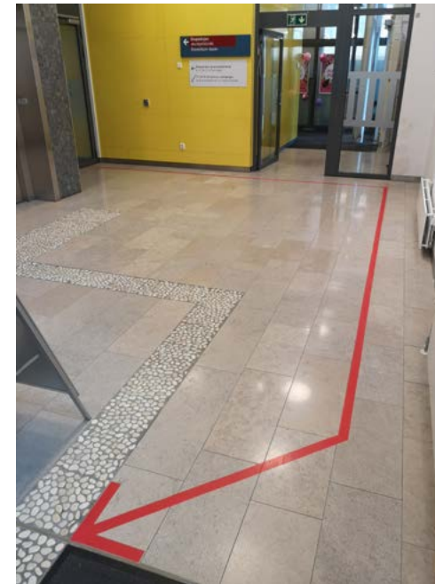
Figure 27: Implementing guiding line on the ground floor leading to the stairs.
