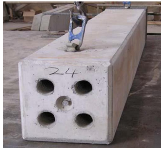
Figure 9: Precast element with coupling sleeves (Volkov, 2019).
