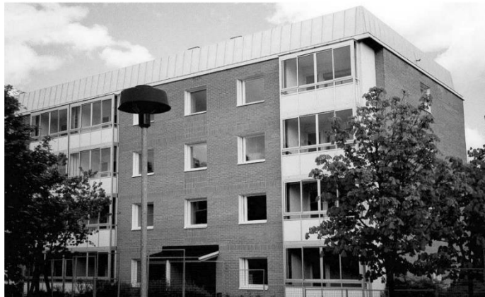
Figure 6: One of the two donor buildings in Finspång before demolition (Eklund, Sundbaum and Ab, no date).
