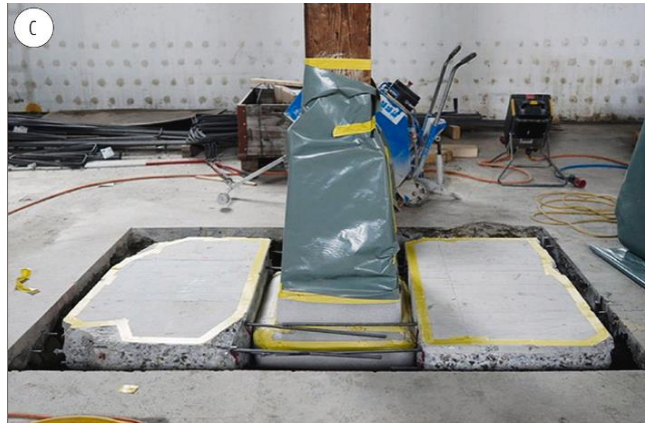
Figure 8: Point foundations of reused concrete blocks (Küpfer, Bastien-Masse and Fivet, 2023).
