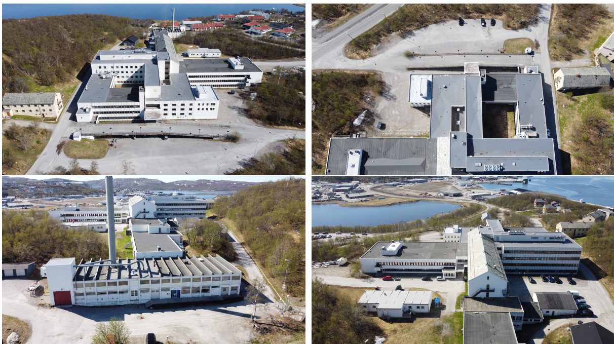
Figure 4.2: The available roof space for the solar panels
