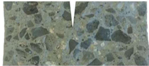
c) Flexural crack
