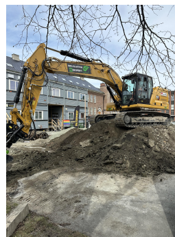
(b) The electric construction machine.
