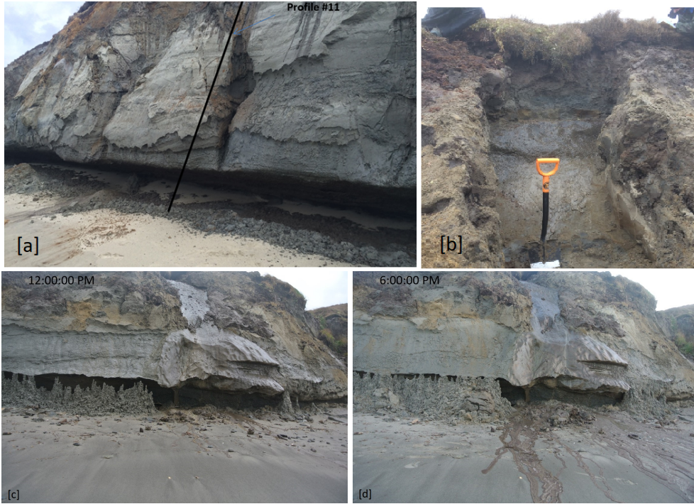
Figure 4.6: [a] Status of Profile#11 during the 2015 measurement. The coastal profile#11 is shown as a black line. A wave-cut niche is visible at the base of the bluffs. Image source: (Isaev et al. 2016) [b] Permafrost inside the bluff was excavated during the field investigation in 2015. Image source: (Isaev et al. 2016), [c,d] six-hour time-lapse of thermodenudation in S#1. Niche is visible at the base of the bluffs, but the bluffs are stable. Accumulation of slumped sediments at the base. Image source: Vladislav Isaev. SAMCoT Report, 2015.
