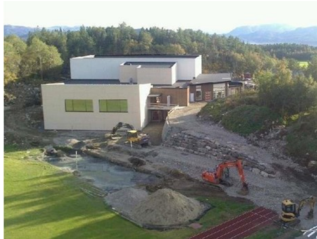
Figure 3. The northern façade of the building.
