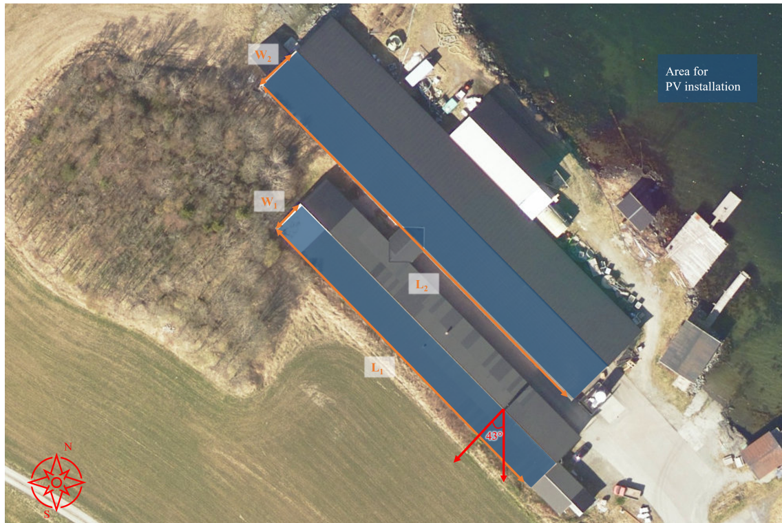
Figure G.2: Overview of the area (roof) that is available for PV modules.
