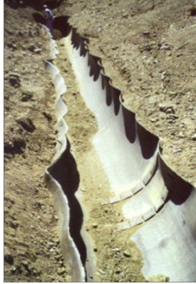
Figure 1.1.: Image of a pipe from a fracture propagation test in [8]. Note that there is a person standing inside the pipe in the upper left of the picture, giving a sense of the scale of this fracture. The image is included with the permission of Xian-Kui Zhu.
