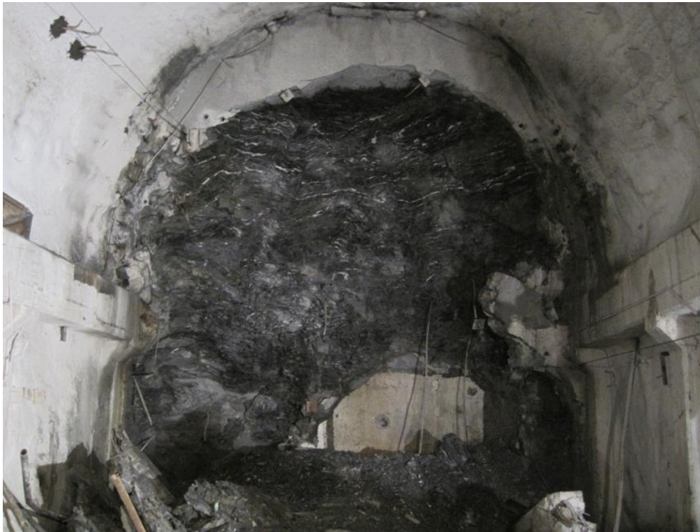
Figure 4-5: Powerhouse cavern after first step of excavation
