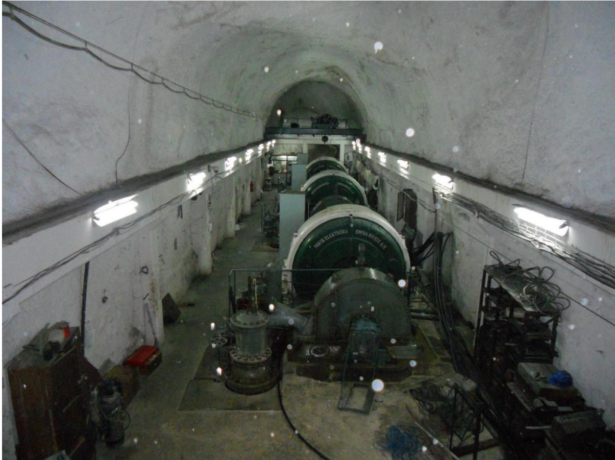
Figure 5-1: AKHP Powerhouse cavern before upgrading
