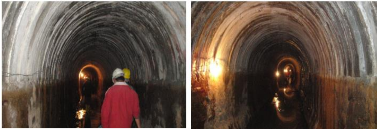
Figure 5-2: Existing tailrace tunnel before the enlargement
