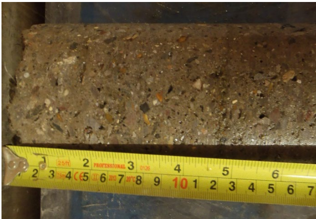
Figure 11 – Photograph showing typical core taken from sprayed concrete lining (photograph Nicholas Trussell)
