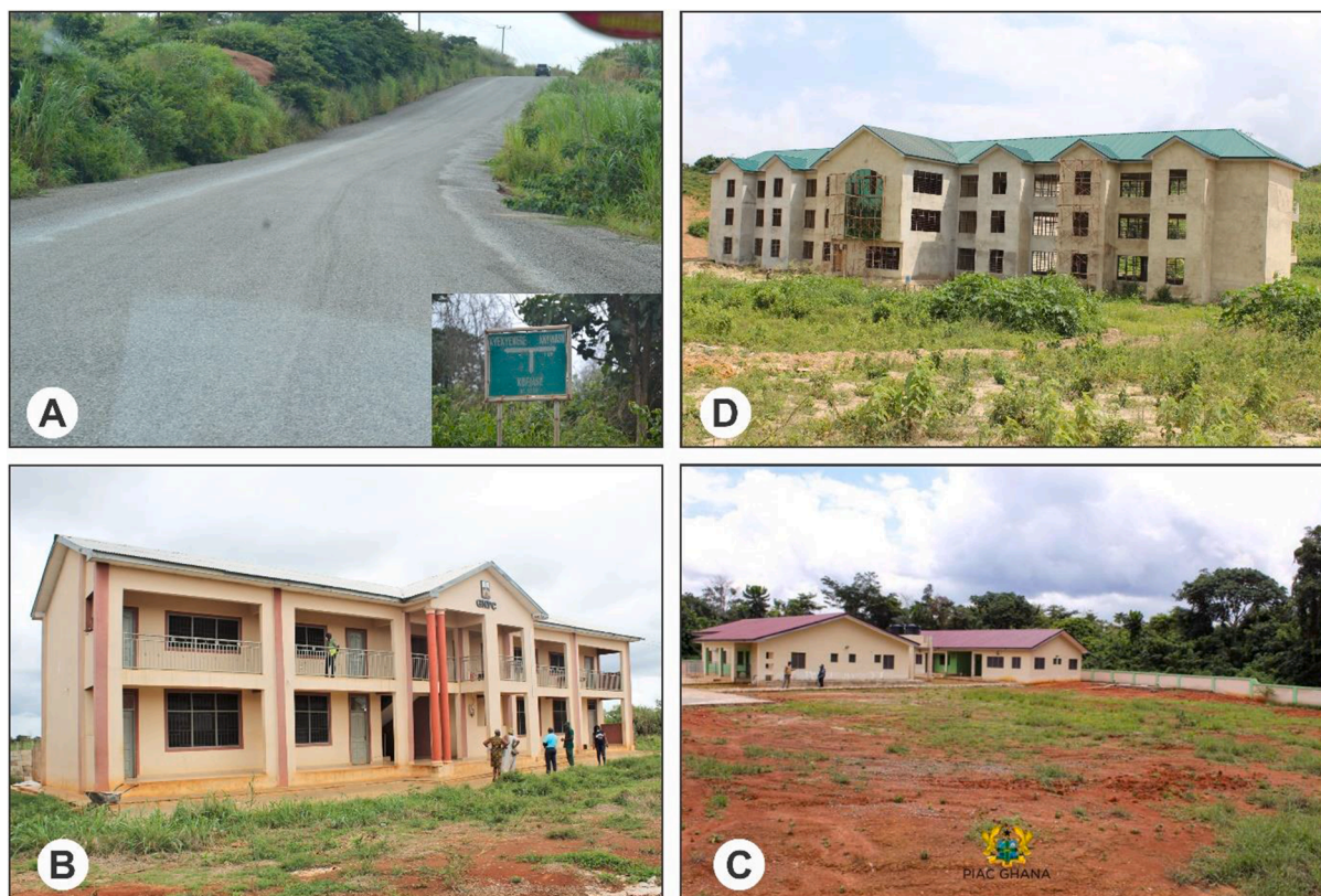
Fig. 2. Some ABFA-funded projects. Notes: The pictures are from PIAC's Facebook page ( https://www.facebook.com/PIACGhana ). A) Anyinasu-Sekyeredumase road in the Ashanti Region. B) Hostel facility (80-bed capacity) in Duayaw Nkwanta in the Ahafo Region. C) Community-Based Health Planning and Services compound in Ahankrasu in the Eastern Region. D) Anomabu Fisheries College.
