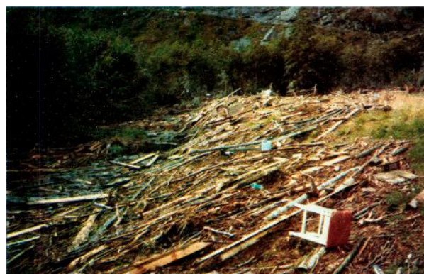
Figure 60: Damaged land near Myklemyr after 1979 flood (Photo: NVE, 1981)
