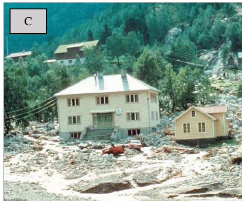
Figure 52: Damage left behind by 1979 flood at Sagrøy: A) Remains of Høgebru bridge (Photo: NVE, 1981), B) Sagrøyelva flowing through building basement (Photo: NVE, 1981), C) Damage left behind by Sagrøyelva (Photo: Hoel, 2013)
